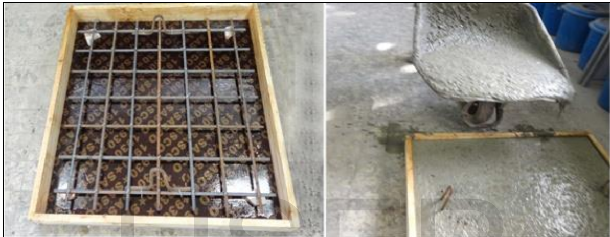
Fig. (2): Casting of slabs.
